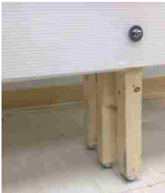
Figure 40 - Single ball caster for each panel's leg
